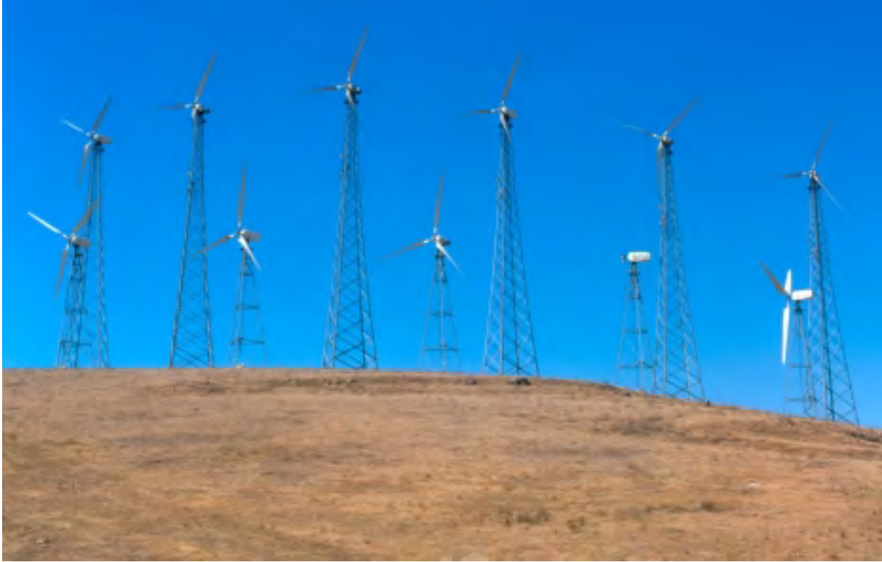
Figure 18. A Windwall consisting of a Row Type-13 Turbines and another row of the Taller Type-23 Turbines (photo by Daniel Driscoll)
